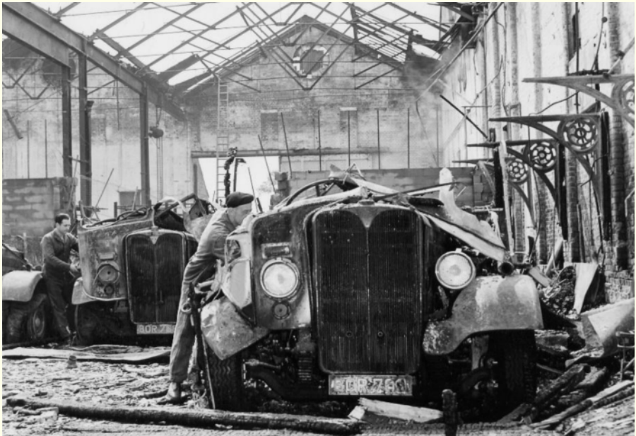
A view of the old East Wing of Hoeford on 18 June 1957 in the aftermath of the Garage fire. No. 37 is nearest the camera with No. 36 behind it.
