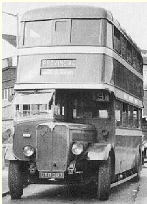
Above: No. 63 (CTO 387) at Gosport Ferry. A unique feature of this bus in the Provincial fleet, was Nottingham's fitting of a route number box between the upper front windows, although this was not used by Provincial. Photo: Stephen Didymus Collection
