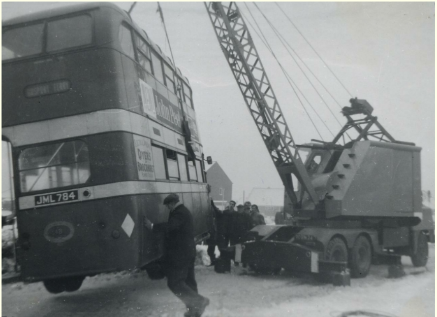
48 about to be placed back onto the road by the Royal Navy crane.
