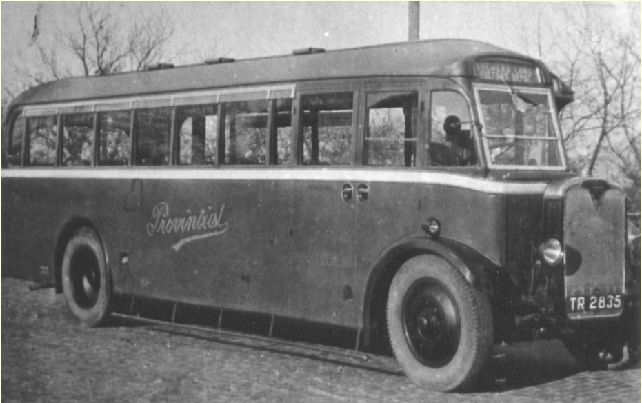
In the late 1930s, Provincial rebuilt the bodywork on some of the former Hants & Dorset Lions to look similar to the AEC Regals which the company operated. Fleet number 6 (TR 2835) is seen here after rebuilding. The earliest withdrawals of these vehicles took place in 1942 and the last withdrawals occurred in 1945.
